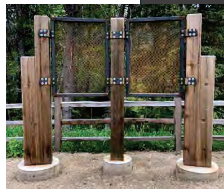
Signage structure at Crescent Valley Beach
